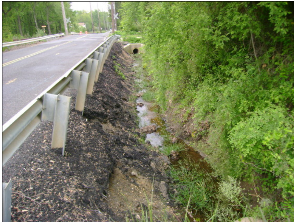
Figure 40. Tributary and culvert at station #45.
