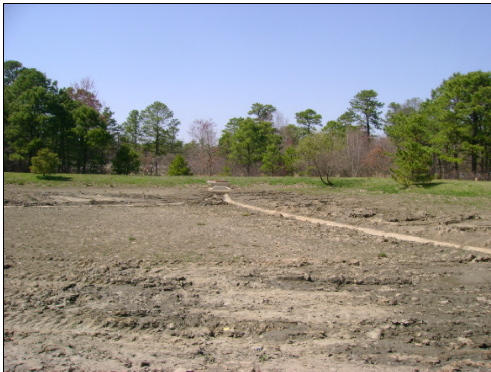
Figure 39. Recently cleared detention basin at station #15.
