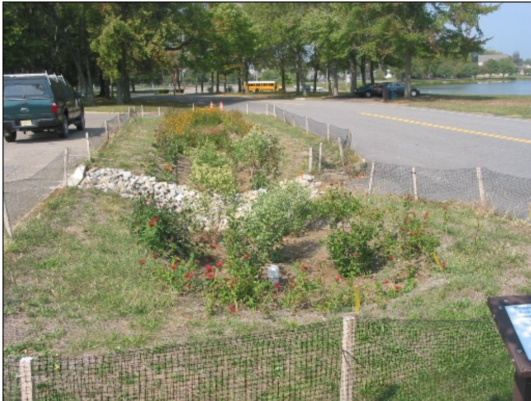
Figure 51. Completed rain garden in August 2010, photo by Rick Lear.
