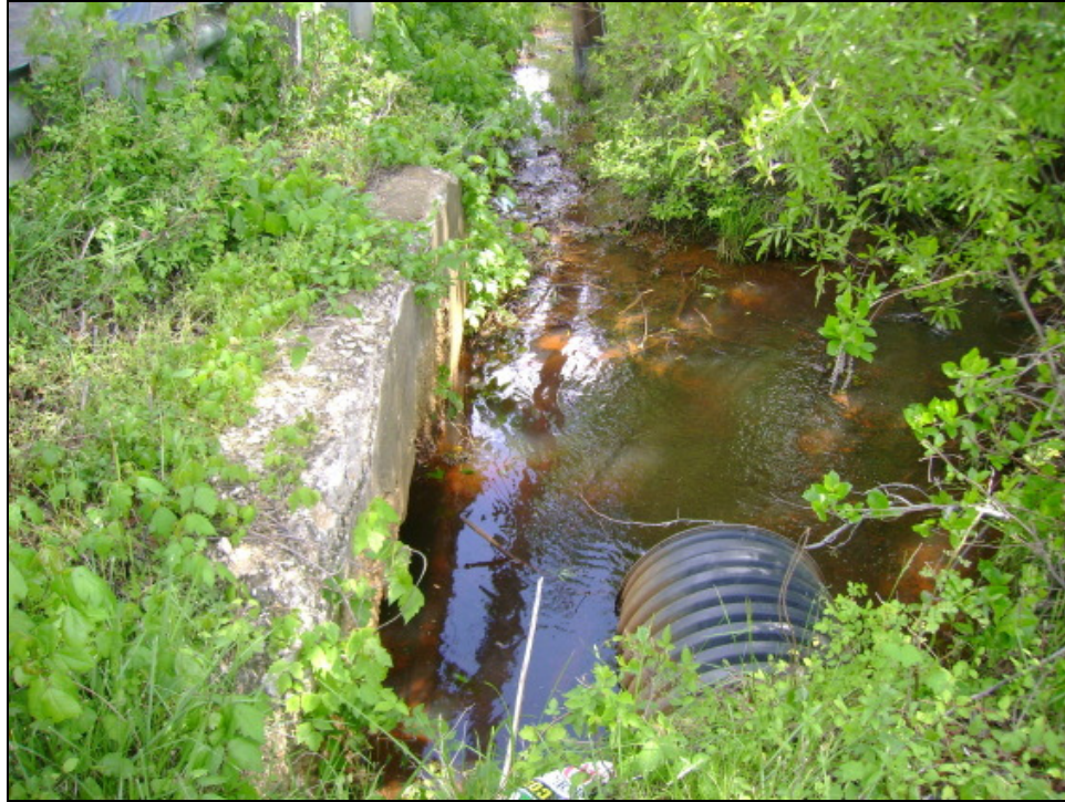
Figure 43. Culvert and swale along Federal Road at station #53.
