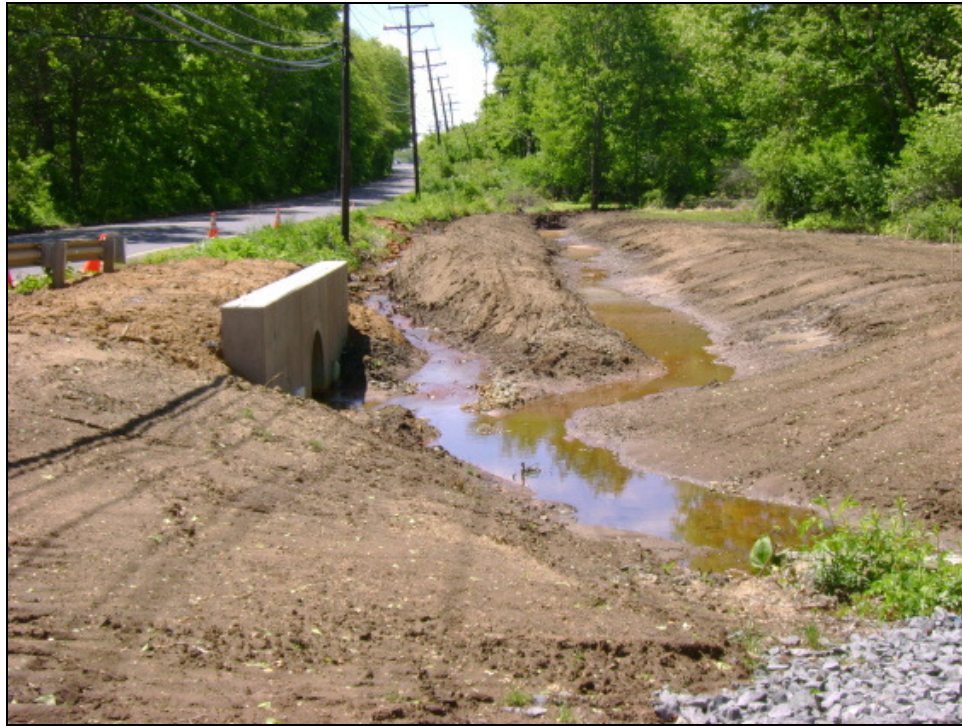
Figure 35. Construction prior to riparian planting at station #71.
