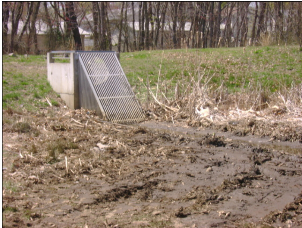
Figure 30. Detention basin outlet structure and recently disturbed vegetation.
