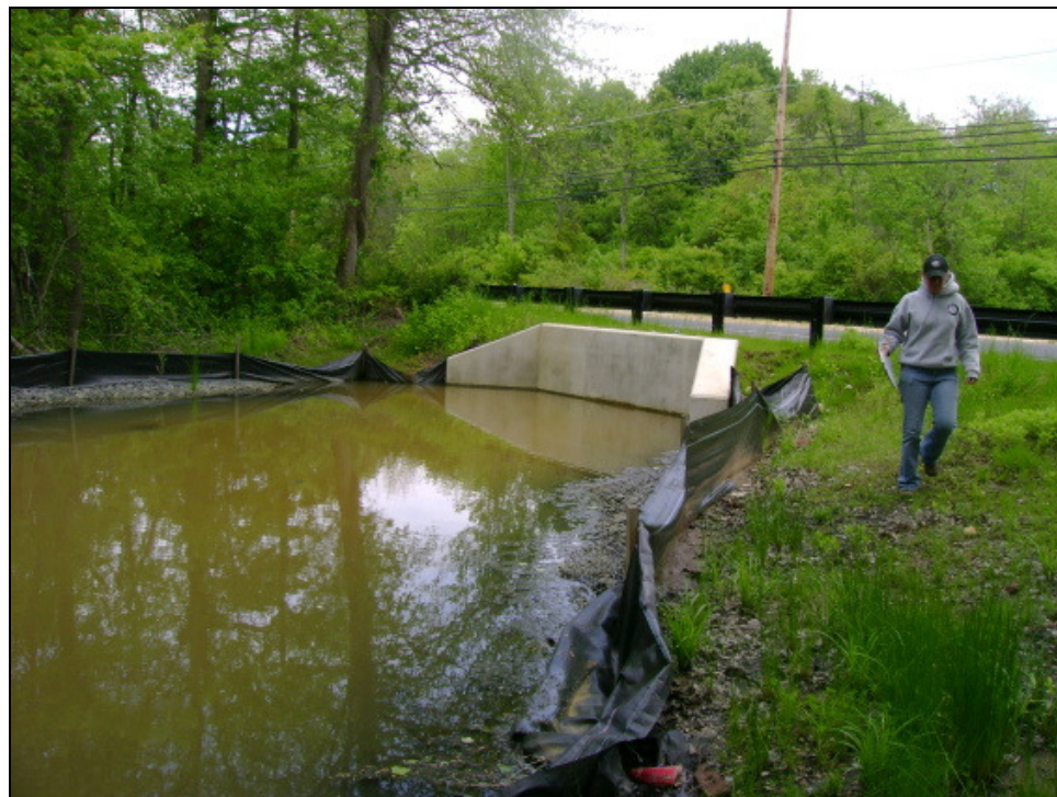
Figure 48. Construction of culvert crossing upgrade at station #63.
