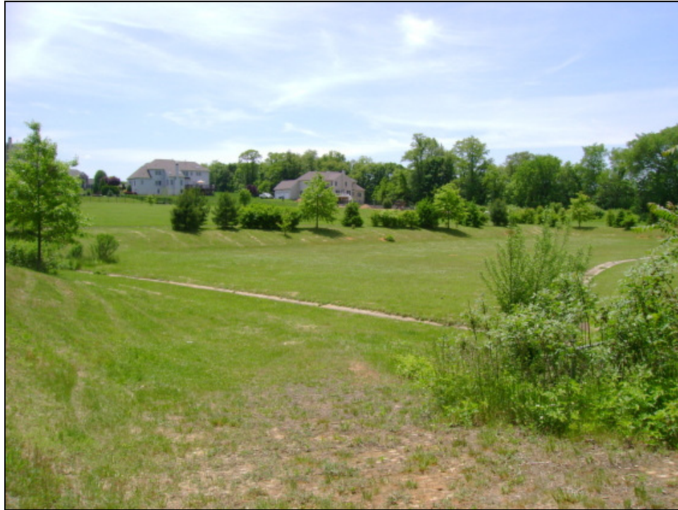
Figure 27. Large stormwater detention basin at station #80.
