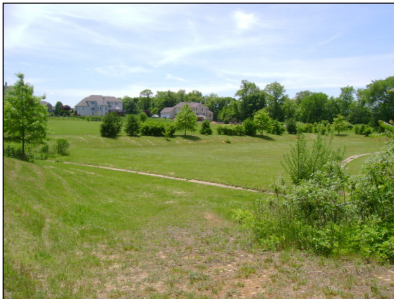
Figure 55. Dry detention basin at station #80, showing turf grass vegetation and concrete low-flow channels, photo taken in summer 2009.
