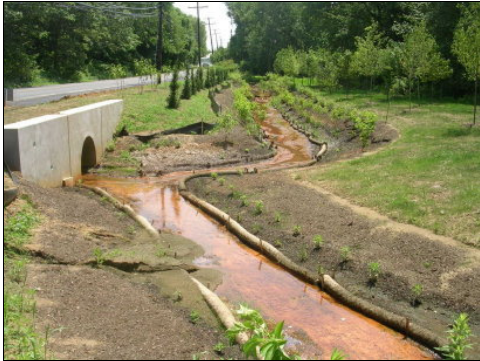
Figure 36. Station #71 after riparian plantings and partial stabilization.
