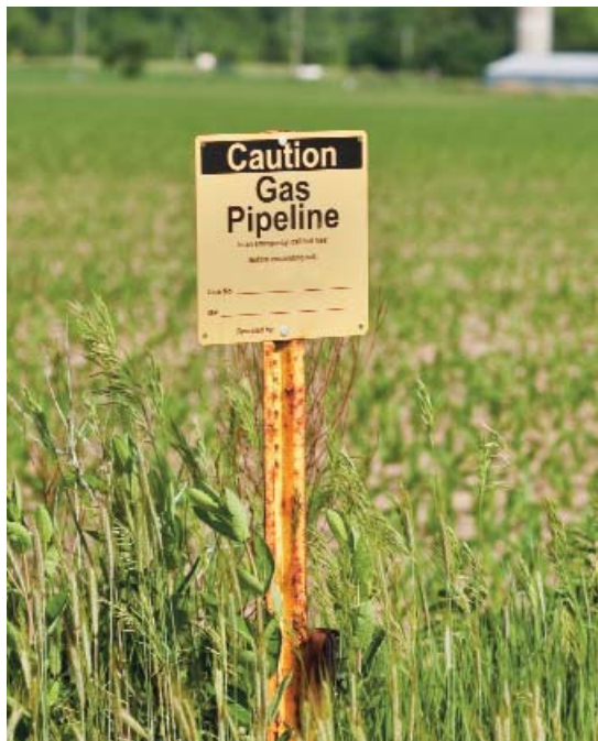
Figure D-8 Underground Gas Pipeline Warning
