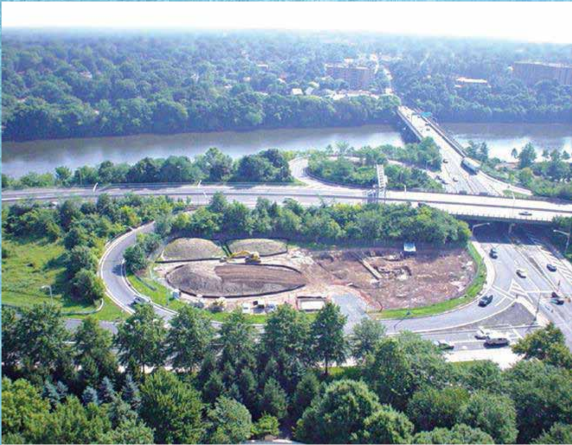
Plate 1. Overhead photograph of Route 18/27 Interchange site from the roof of Johnson and Johnson International Headquarters. Photo by Shane Whilden, 2003. Vol. 1, pg. 25.
