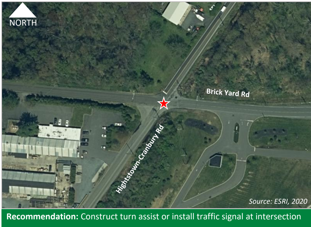
Figure 29: Hightstown-Cranbury Road at Brick Yard Road
