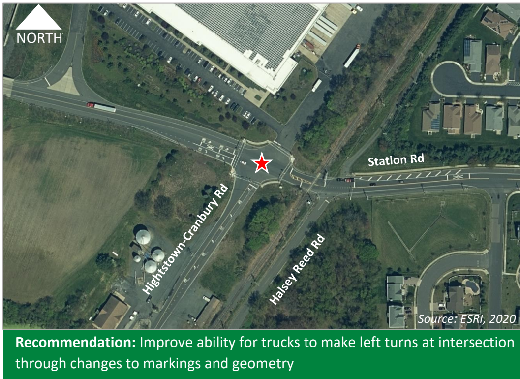
Figure 30: Hightstown Cranbury Station Road at County Route 615 (Station Road)
