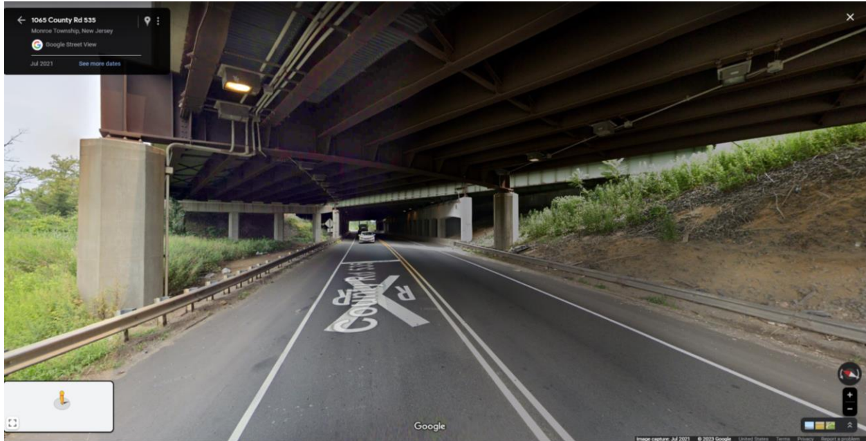
Figure 38: CR 535 (Cranbury-South River Rd) below New Jersey Turnpike (looking north)
