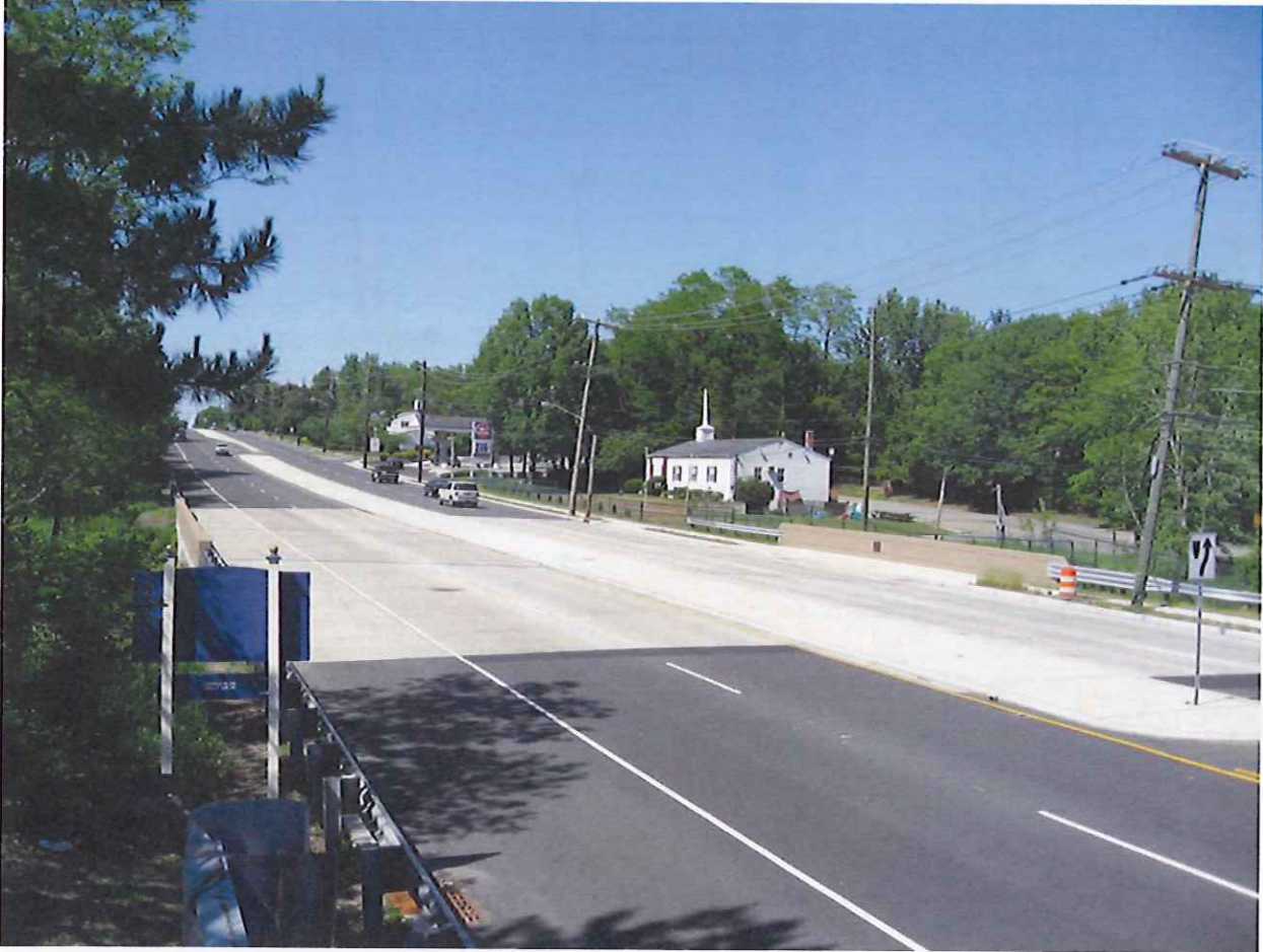
Ryders Lane Bridge over Saw Mill Brook
