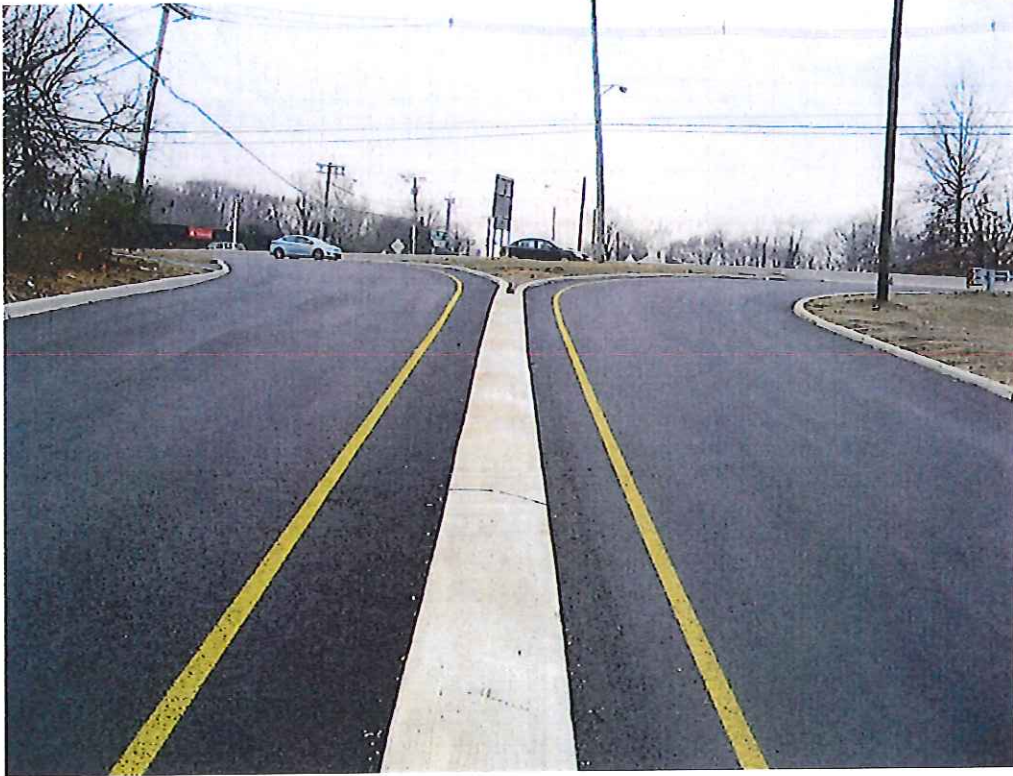
Route 9 Ramps Repaving Sayreville Borough
