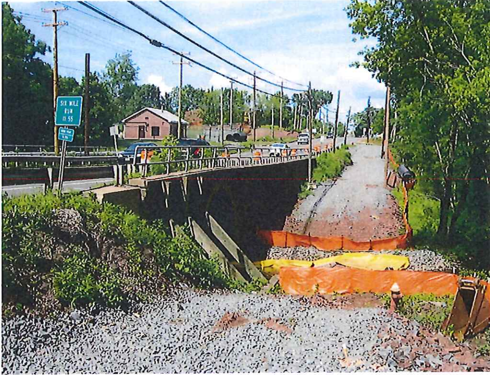
NJ Route 27 Bridge over 6mile run North Brunswick Township
