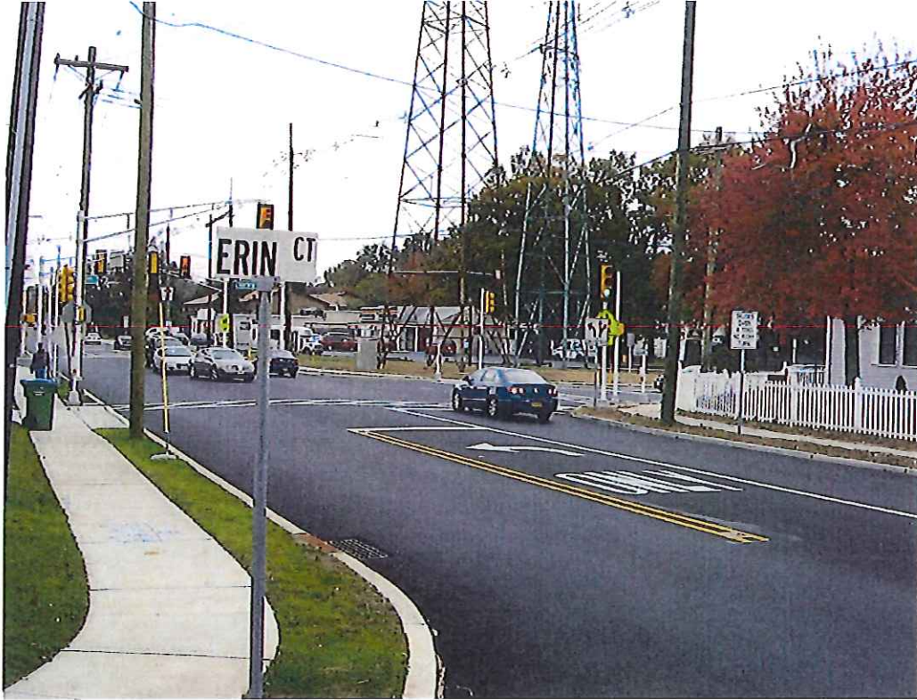
CR 514/Woodbridge Avenue – Gurley Road – Trenton Avenue Intersection Improvements Edison Township
