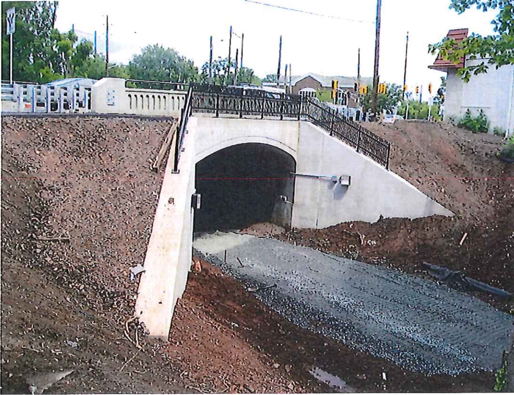
NJ Route 27 Bridge over Middlesex Greenway Metuchen Borough
