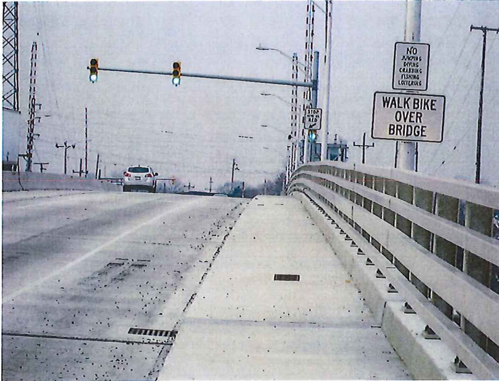
NJ Route 35 Draw Bridge over Cheesequake Creek Old Bridge Township
