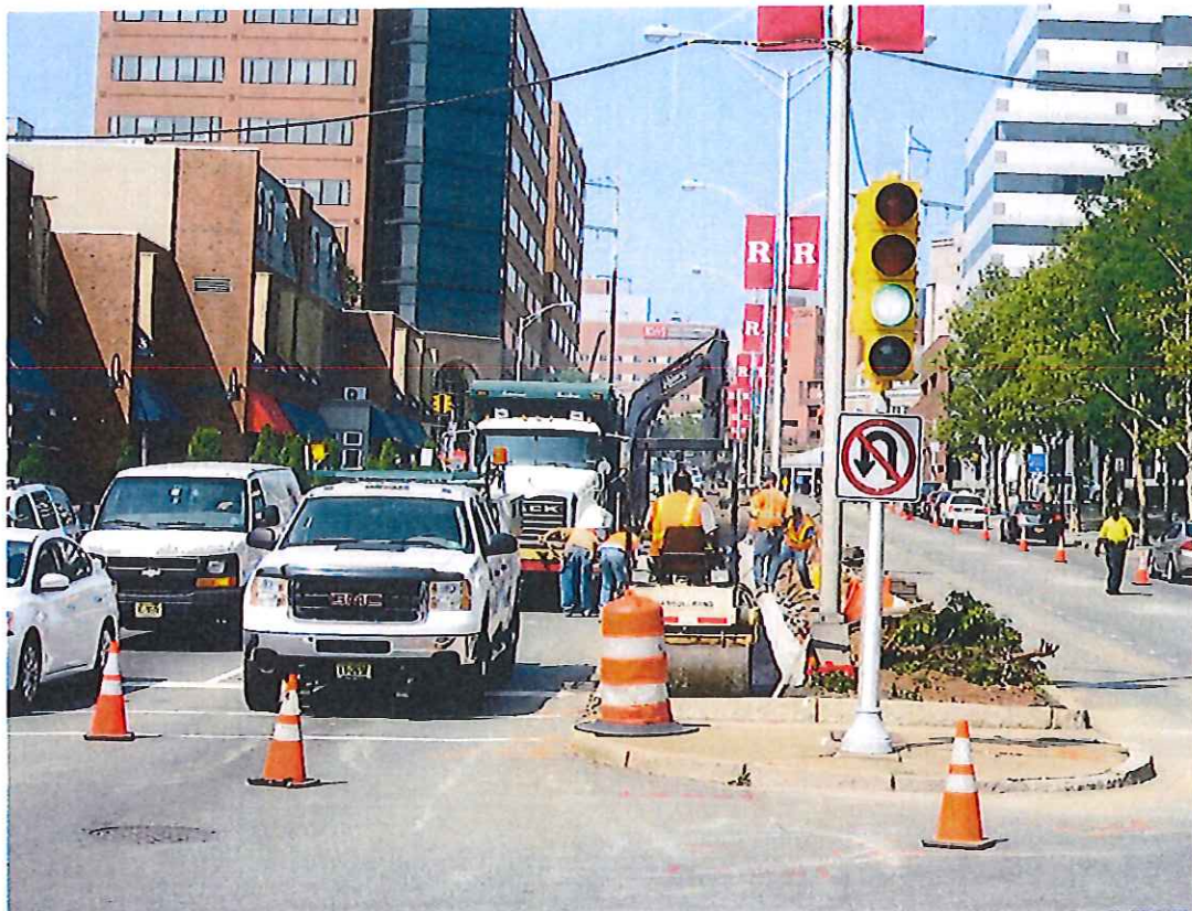
Route 27 at Nielson Street – New Brunswick Bikeway Construction New Brunswick City
