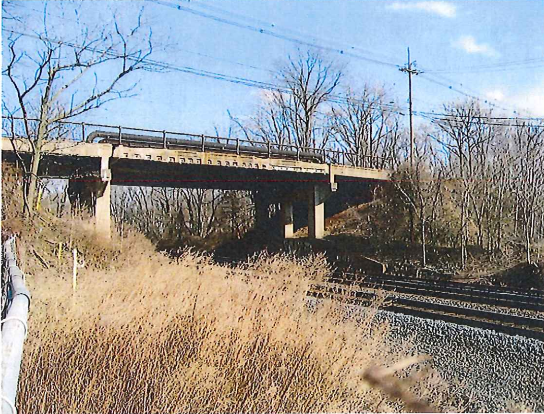
Park Avenue Bridge over CSX South Plainfield Borough and Edison Township
