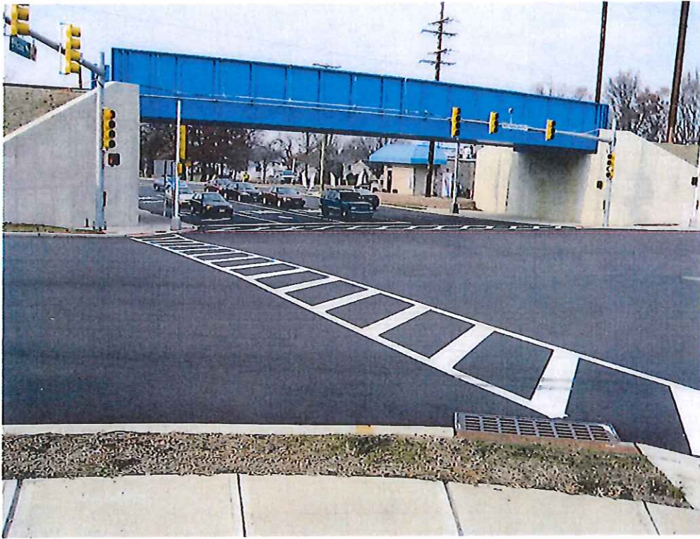
Ernston Road & CSX underpass at Bordentown Old Bridge Township & Sayreville Borough
