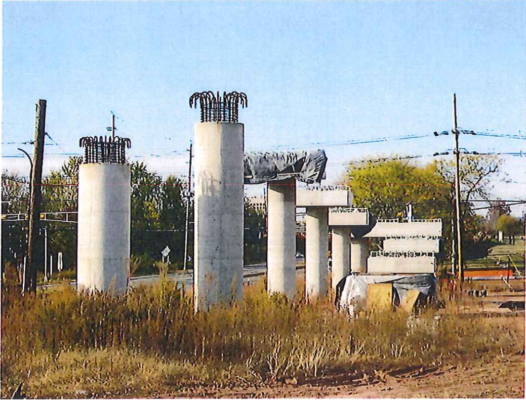
NJ Route 18 Extension Pedestrian Overpass Piscataway Township
